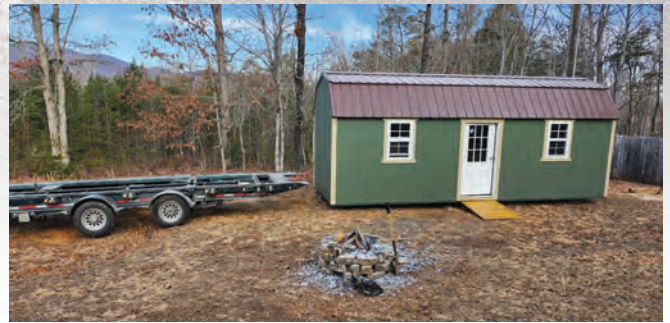
The sheds don't have running water, and are dependent on generators for power, when fuel is available, but they're a welcome relief from tent camping.
