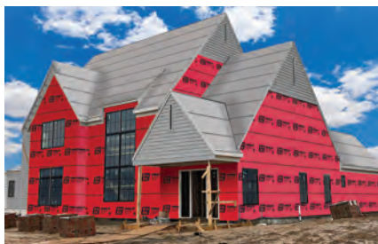
Grip-Rite's ProWrap SA is a timesaving, self-adhering wrap that reduces labor that's rated for both residential and commercial applications.
