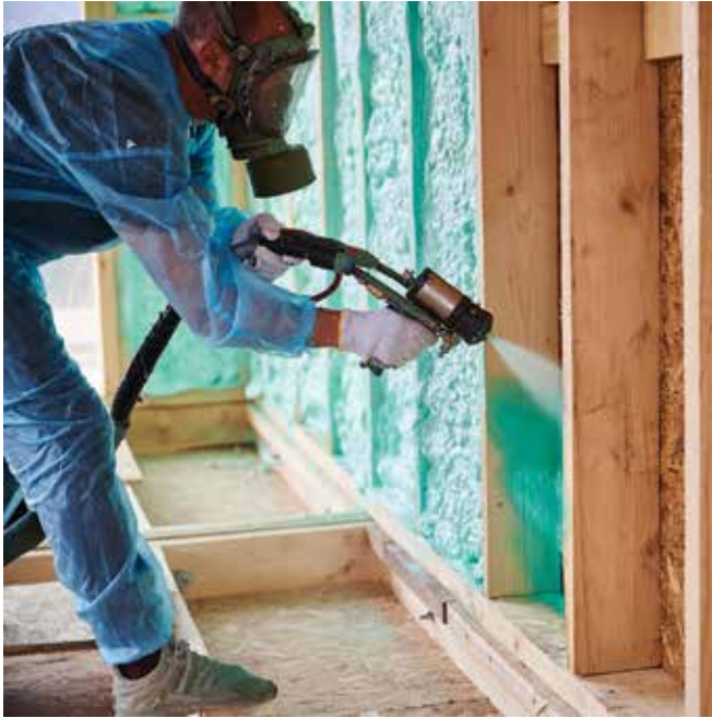
Spray foam insulation.
