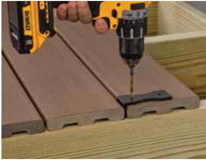
FastenMaster's hand alignment guide for aligning fasteners on scalloped decking.
