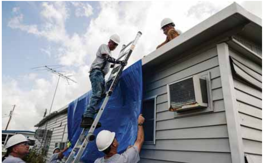
Hurricane response in Florida.
