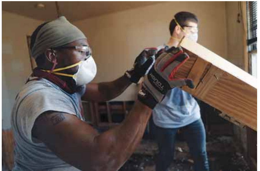
Rebuilding in Selma, Alabama.
