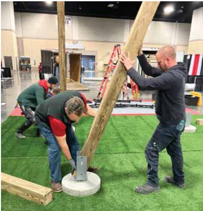
The first post is set into a post bracket.
