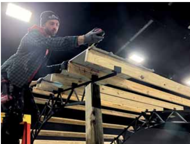
Prefab steel trusses are manufactured to precise specifications, ensuring a smooth assembly process compared to wood trusses.
