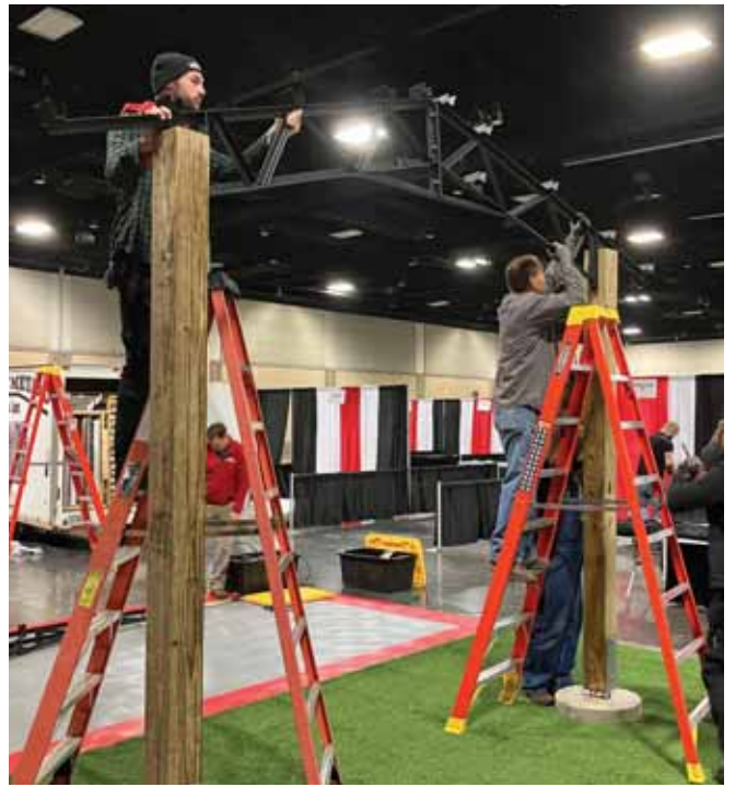
Steel trusses are immune to rot and insect damage that can shorten the lifespan of wood trusses.
