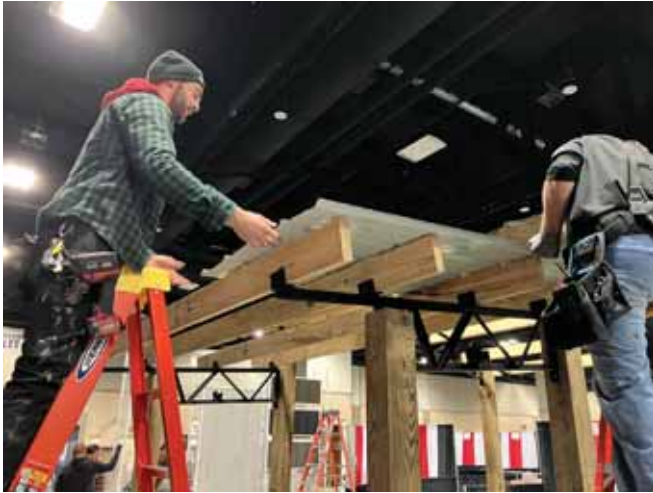
Although a steel truss is more expensive than a wood truss, it can take the place of five or six wood trusses, which saves money.
