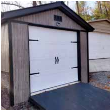
The new shed is next to an existing garage.
