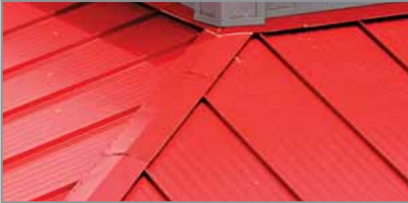
Two very different metal roofing looks. (TOP) Seamed panel in Aged Metal from A.B. Martin Roofing Supply. (BOTTOM) Ribbed-steel roof coated with Sherwin-Williams Coil Coatings' WeatherXL Crinkle Finish..
