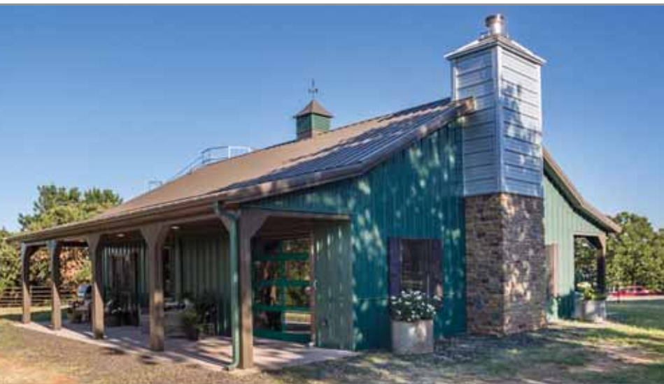
The brown and green color scheme on this post-frame cabin blends in with its surroundings. COURTESY OF MORTON BUILDINGS
