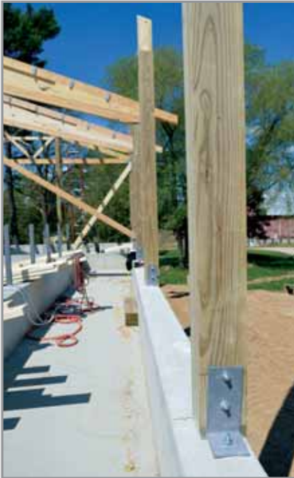
Modern post-frame design prevents rot by keeping wood away from the soil.
