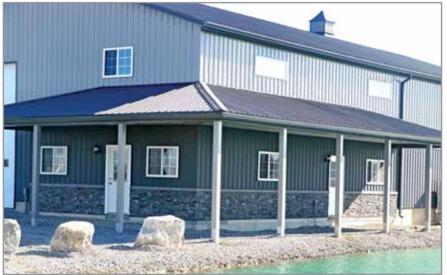
This large post-frame "shouse" features divided-light windows, a cupola, a corner porch, and faux stone URESTONE wainscot. COURTESY OF REPLICATIONS UNLIMITED
