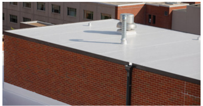
White Liquid Rubber Coating. PHOTO COURTESY OF INLAND COATINGS
