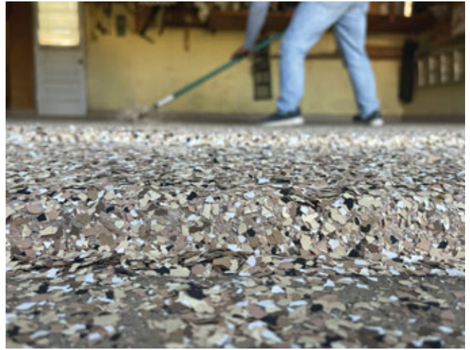
“Large Flake” flooring install.
