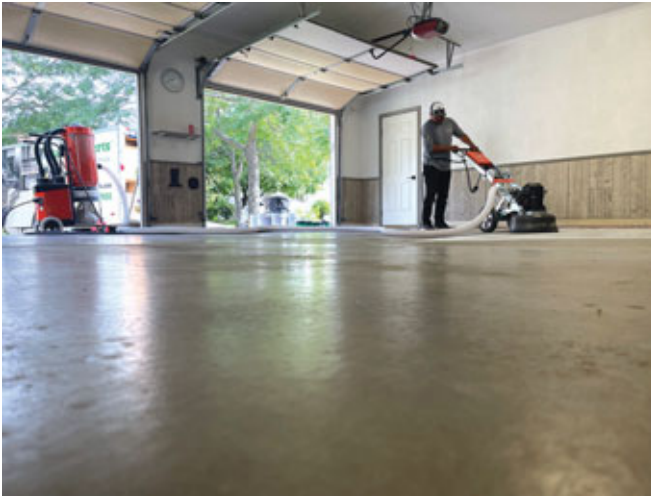
Grinding the floor so the epoxy will bond with the cement.
