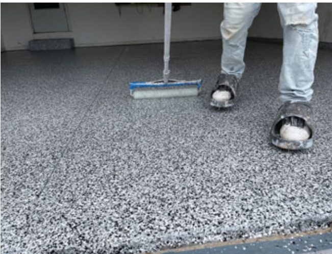
Cleaning the floor is the final step.
