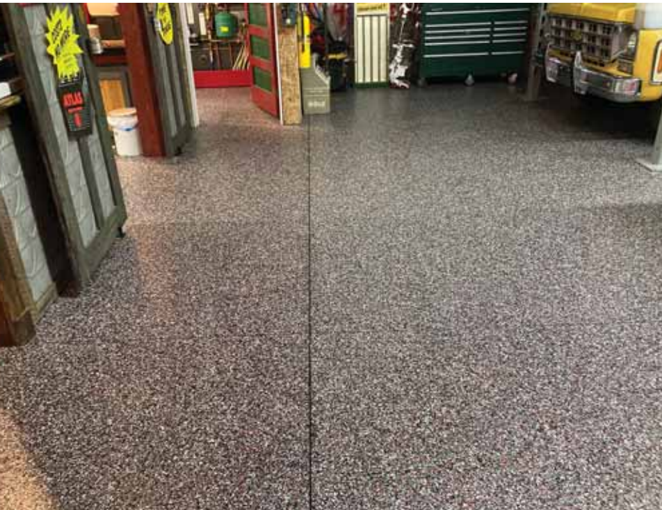
Garage Experts provided the custom flooring throughout. PHOTO BY ANTHONY BRASS
