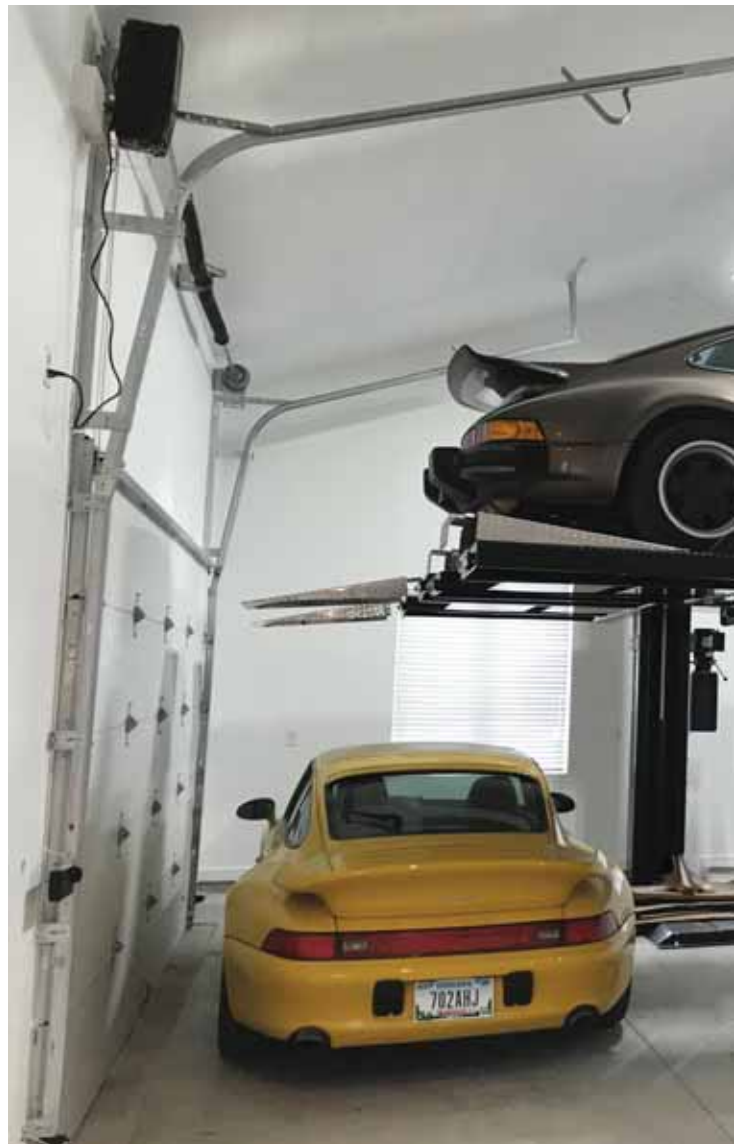
High-lift system with track extended closer to vaulted ceiling allows more cars and headroom between elevated car’s roof and ceiling.
