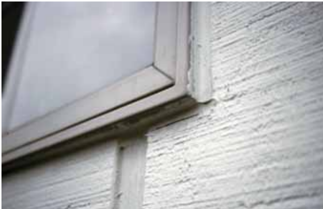
Figure (Pic.) 8—A perimeter sealant joint around a contemporary flanged window. The joint is of appropriate width at 6 mm (0.25 in.). The joint had been in service for roughly 3 years when photo was taken. Joint is mostly intact, but some adhesion failure is evident at lower right corner. As is common in residential construction, neither bondbreaker tape nor sealant backer was used. Joint failure is likely the result of three-sided adhesion, an unprimed siding edge, and other-than-ideal sealant width–depth ratio (sealant depth exceeding width).
