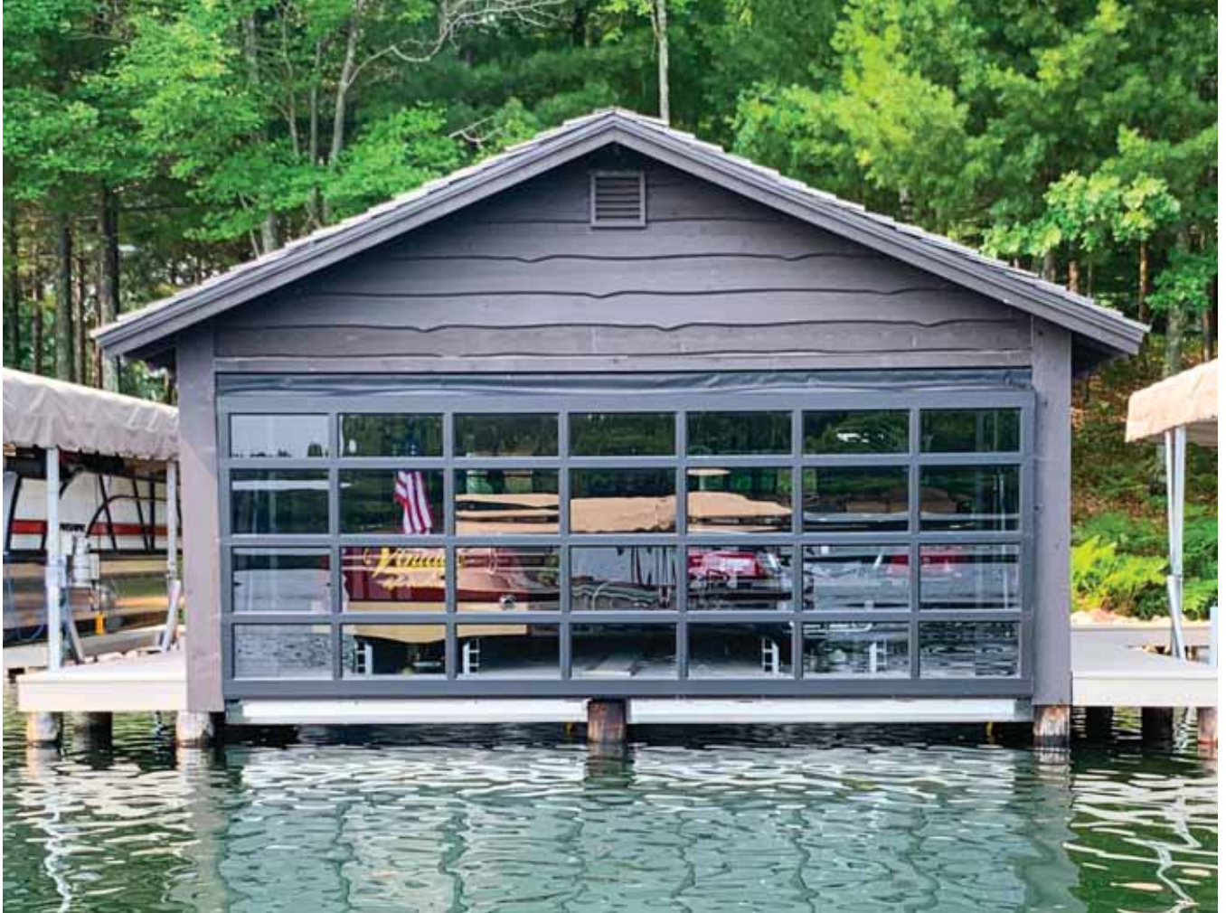
Above and Left: The custom boat house door is a full-glass hydraulic door and extends out. Midland Door Solutions supplied the door. PHOTOS COURTESY OF CENTRAL DOOR SOLUTIONS.
