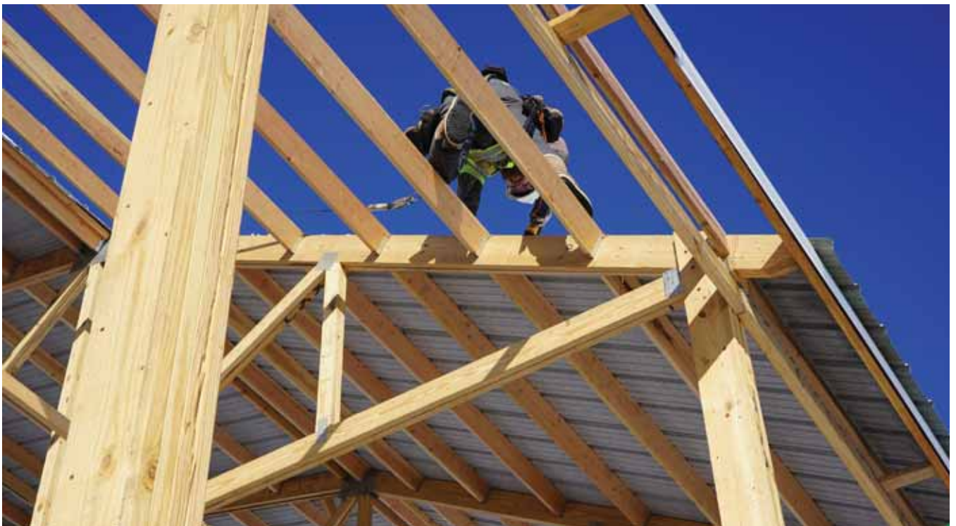
Condensation will form on the underside of cold, untreated roofing panels when warm, humid air rises and hits the metal. Pre-applied membranes absorb the moisture and release it back into the air as humidity. COURTESY OF DRIPSTOP.
