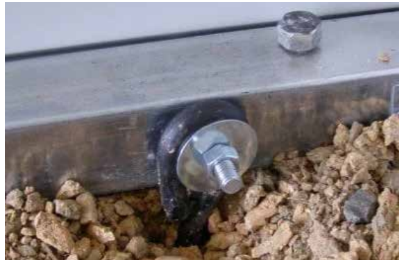
When installed properly, anchors are difficult to see.
