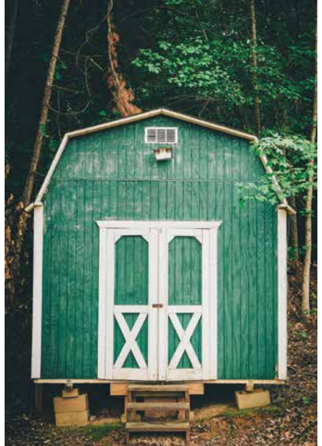
Don't be “that guy” that gives shed delivery and set-up services a bad reputation. Shimming over 12” makes for an unstable shed. PHOTO BY REX WAY/ UNSPLASH.
