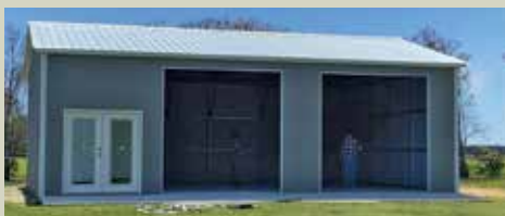
PRE-BUILT STRUCTURES, MT. AIRY, NORTH CAROLINA. PHOTO COURTESY OF NATHAN BEARD, RTO NATIONAL.
