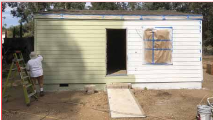
Master painter Mike McSweeney says it takes nine hours of preparation for every hour of painting; he left the paint preparation to Chris Geldert and Mark Pilcher, while he focused on the skilled work of paint spraying.
