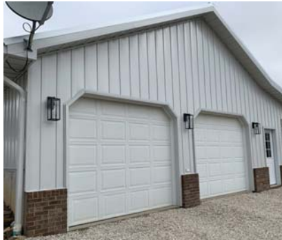
This multi-purpose shed features steel Board & Batten panels from Graber Post Buildings, giving the structure a traditional look. The wainscot is Versetta Stone. PHOTO COURTESY OF GRABER POST BUILDINGS, INC.
