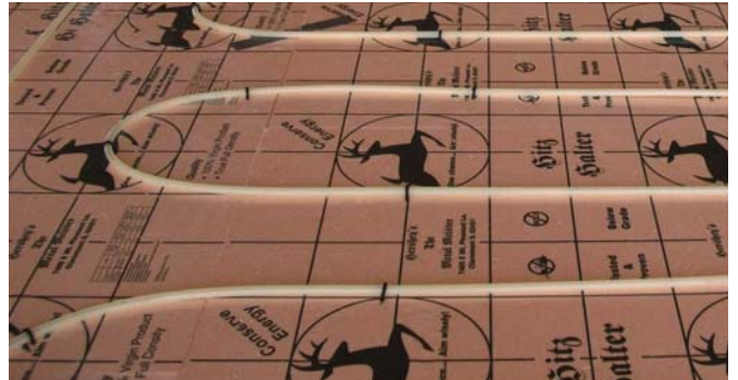
The marked grid makes rebar and PEX tube placement as simple as following the lines.
