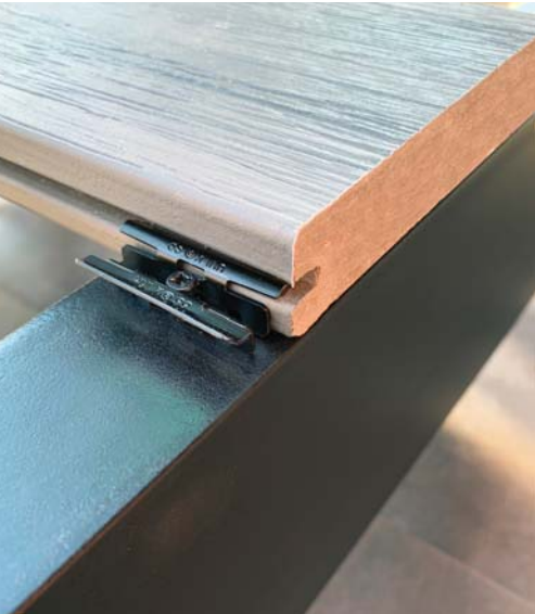
Because contemporary solid-core composite decking can be expected to last for decades, more homeowners are requesting decks built with steel framing. COURTESY OF FORTRESS BUILDING PRODUCTS
