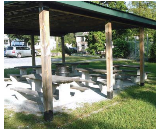
Notches in the buried ends of GreenPosts prevent wind from pulling the posts out of the ground. Up to a 72" barrier can be applied to GreenPosts.
