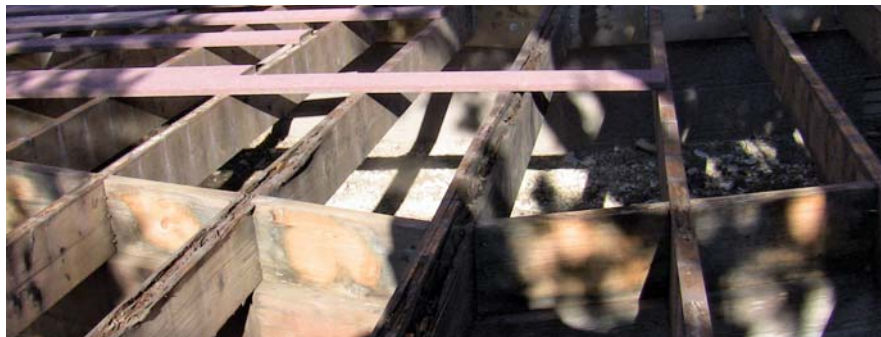
The ledger board and top of the deck joist are sealed, which will help prevent water from causing rot and decay.
