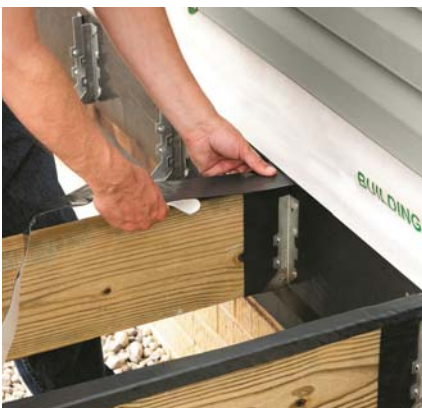
The ledger board and top of the deck joist are sealed, which will help prevent water from causing rot and decay.
