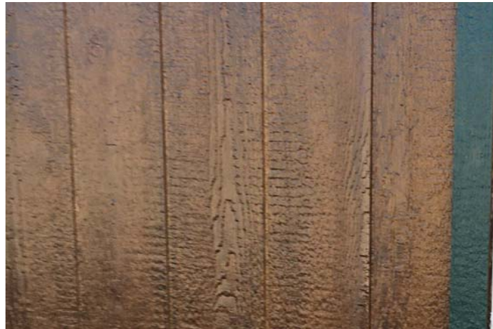
After Chestnut touch-up. The shed was originally coated with PPG Semi-Transparent Chestnut Urethane, and was then touched up with Chestnut Aerosol.
