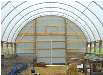
Plenty of light and ventilation make a fabric building well suited to animal confinement.
