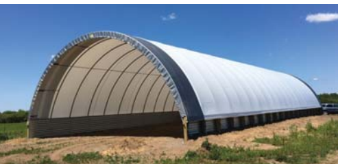
A crew of three to five will have no trouble setting up a single-tube ProTec structure.
