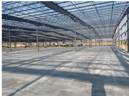
The building of Wausau Supply Co.’s Butte, Montana, warehouse is in progress.
