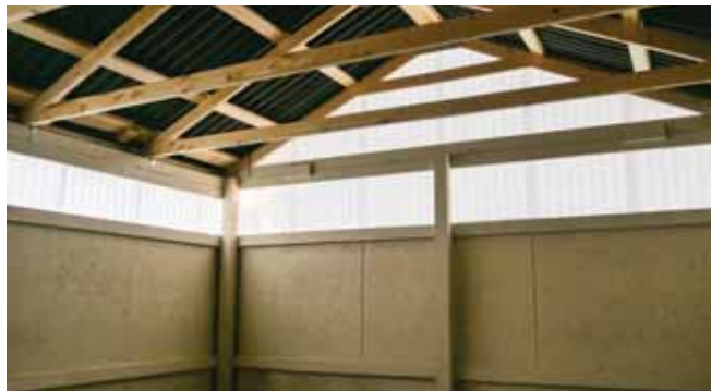
TUFTEX corrugated polycarbonate panels allow up to 90% light transmission and are 20 times stronger than 5 oz. fiberglass corrugated panels. PHOTO COURTESY OF ONDULINE.
