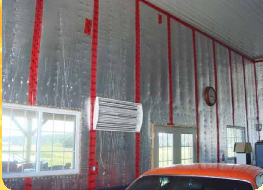
The double-faced reflective foil insulation in this shop will make it a whole lot easier to heat and cool. Note the taped seams to prevent heat and moisture transfer. PHOTO COURTESY: COVERTECH
