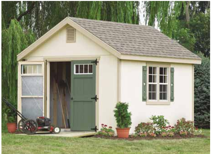
Including gable vents in a garden shed prevents VOC buildup and results in a healthier work and storage space for the owner. PHOTO CREDIT: LOUISIANA PACIFIC
