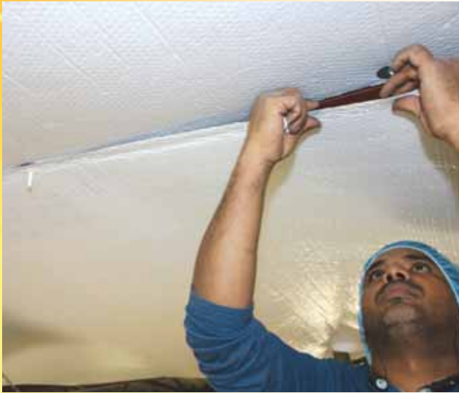
Installing foil insulation with rFoil's Retrofit MBI System. PHOTO COURTESY: COVERTECH
