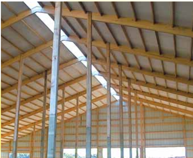
Covertch's rFoil installed between the roof panels and the purlins on this post-frame structure will keep the building considerably cooler during hot weather. The ultimate goal in an un-conditioned building is to match the inside temperature to the outside temperature. PHOTO COURTESY: COVERTECH
